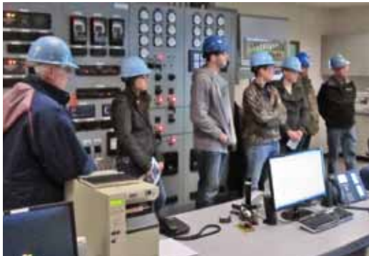
The Junior Board was allowed to tour the control room at the plant.
