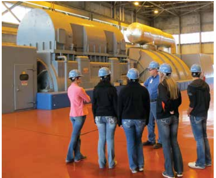
The five members of the Lane-Scott Junior Board learn about the generating turbine at Holcomb Station.
